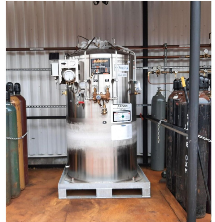
Microbulk gas storage tank.
